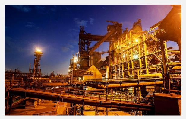
The blast furnace shell integrity and geometry were restored, bell-less top was replaced. The whole furnace shaft relining was done with BAT and refractory lining of hearth and hearth bottom was recovered.
