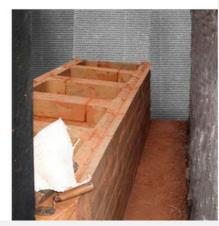
«Hot repairs» with partial cooling of repaired vertical flues and other oven areas
