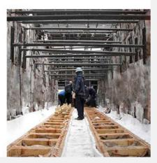
«Hot repairs» with partial interruption of heating and cooling the brickwork of adjacent heating walls group
